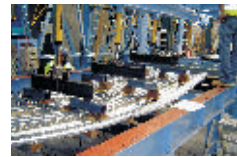
Formwork - Point Load
